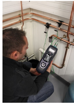
DHW network temperature
