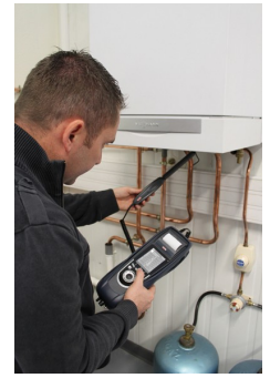
Ambient CO checking
