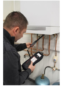
Ambient CO checking
